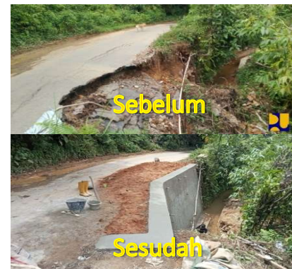
Gambar 2 Dinding Penahan tanah
